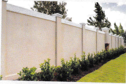
Wall Compound to Entire Layout
